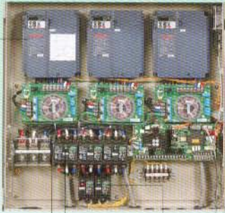
Earth leakage circuit breaker
